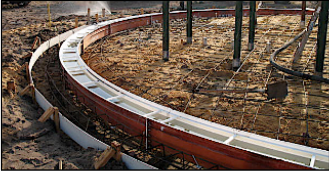
The preferred modular fiberglass gutter system for rimflow pools, zero entry, beach entry and spray deck designs.
